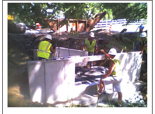
Installation of the endwall for the S. 32 nd Street culvert.
