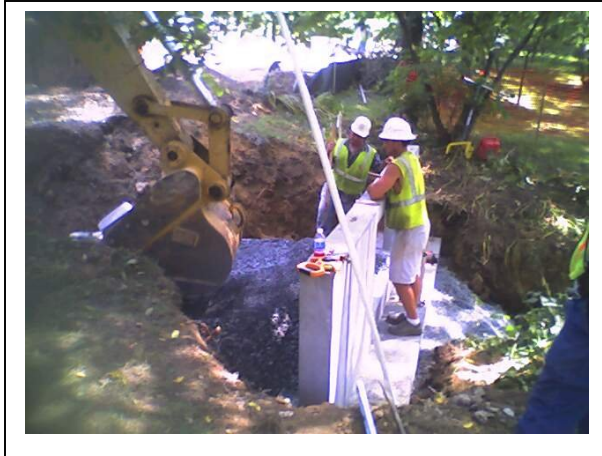
Installation of the endwall for the S. 32 nd Street culvert.
